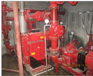
Photo of fire safety equipment Fire Pump.jpg
