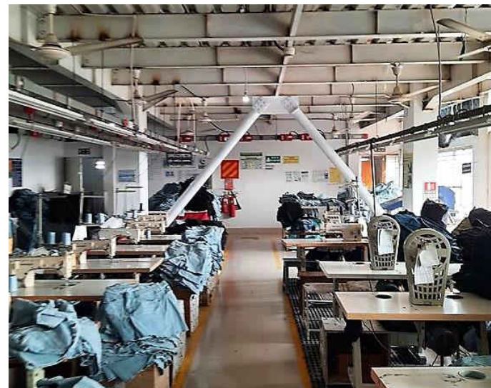
Inverted V Bracing at 3 rd floor
