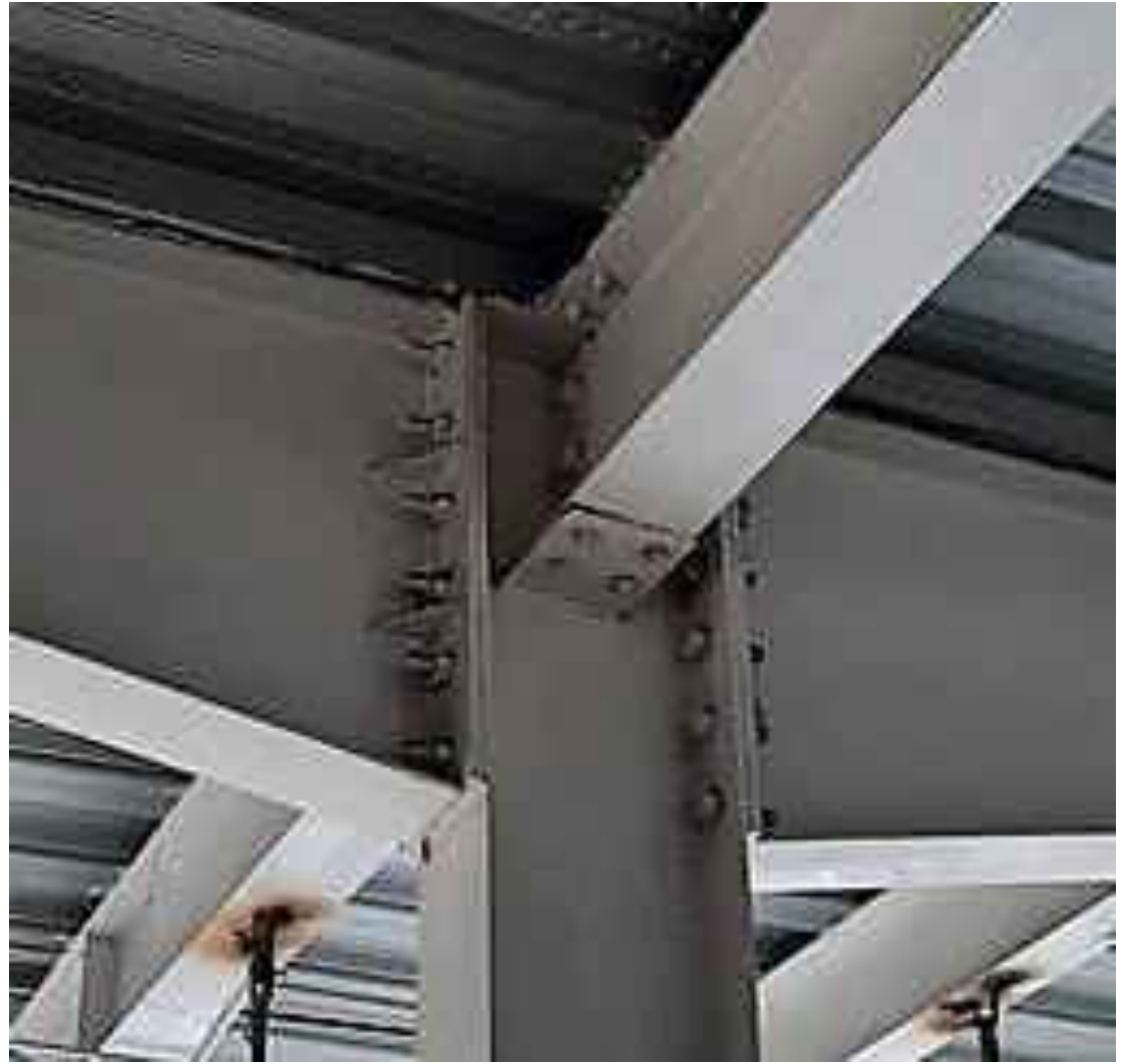
Column-Main Beam- Sub Beam Connection
