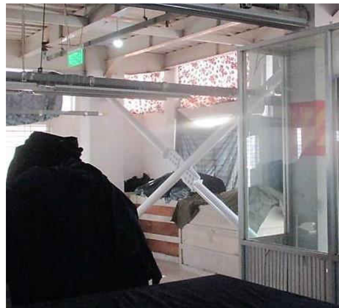
Cross bracing at 4 th floor
