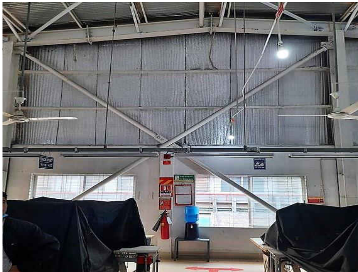
Cross bracing at 1 st floor
