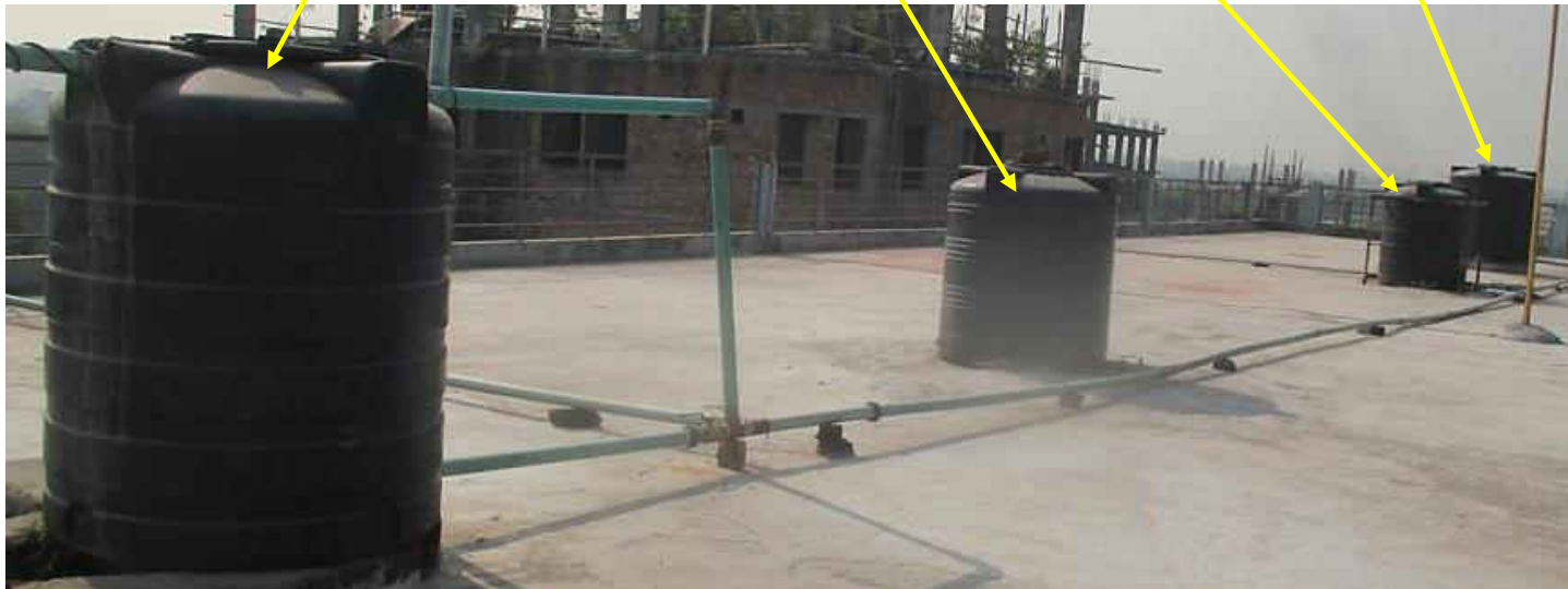
Plastic water tanks on roof top
