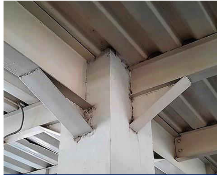
Beam-Column Joint
