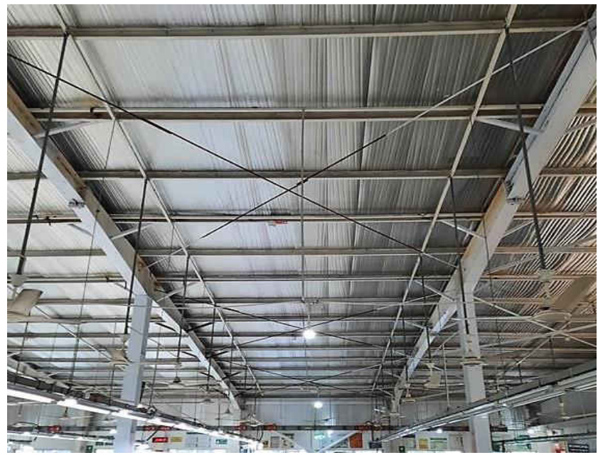
Cable bracing on roof
